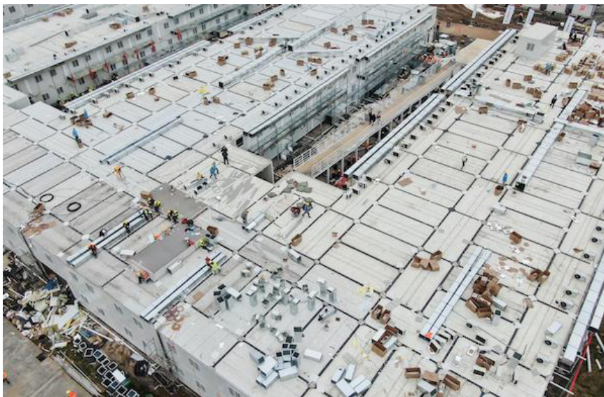
Figure 3-9: Assembly of container-type mobile wards (provided by CSADI)
