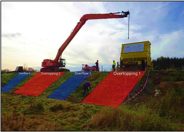
Figure 1. Overview test locations on embankment.
