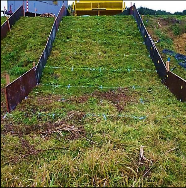
Figure 3. Overview picture taken prior to the first wave overtopping experiment
