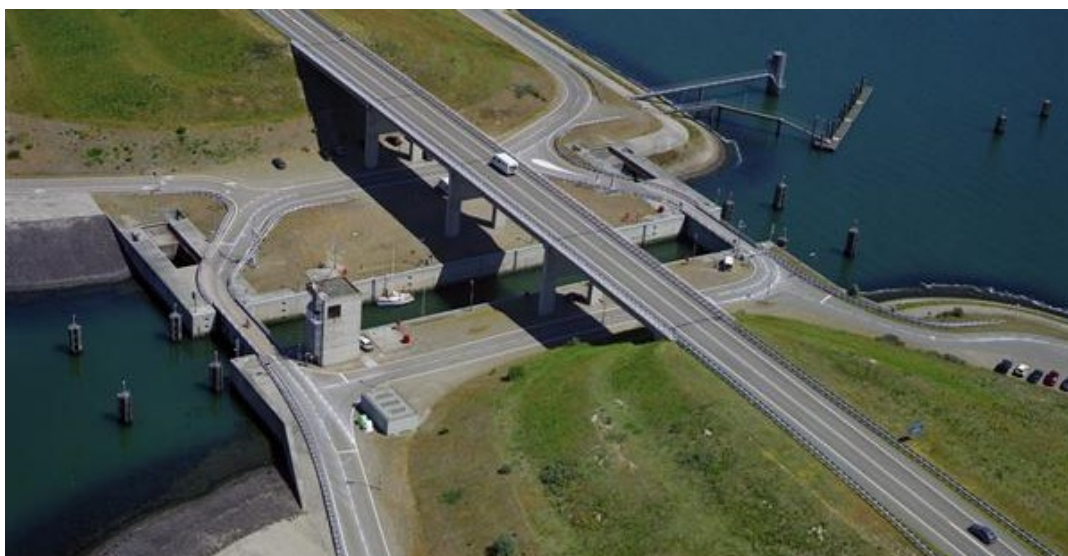
Figure 2.8: An aerial photo of the Roompotsluis, [50]
