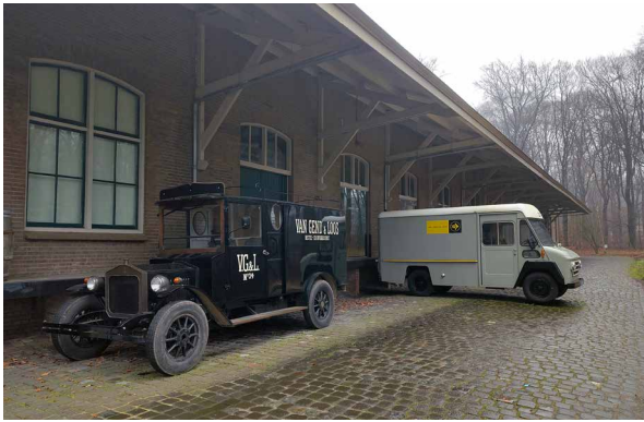
FIG. 2.30 Van Gend & Loos warehouse Tiel, built around 1900, currently in the Dutch Open Air Museum Arnhem. Photo: Merten Nefs.
