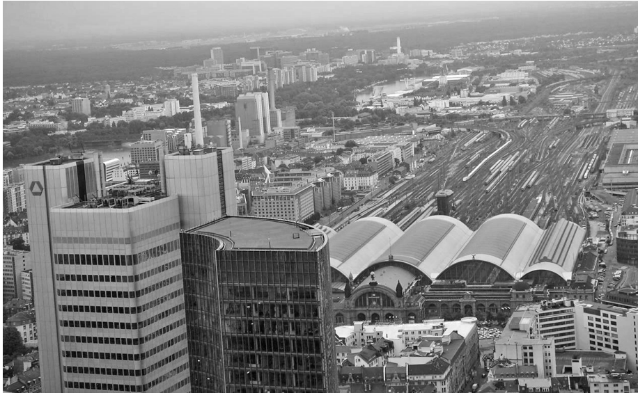
Figure 4.1 High-speed train station in Frankfurt
