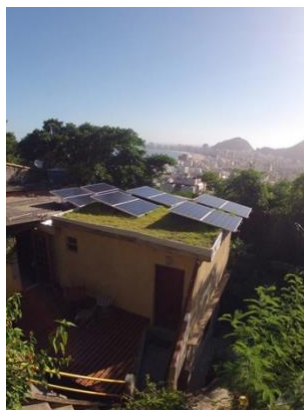
Figure 13. “Estrelas da Babilônia” PV power plant (2016). Source: Revolusolar .
