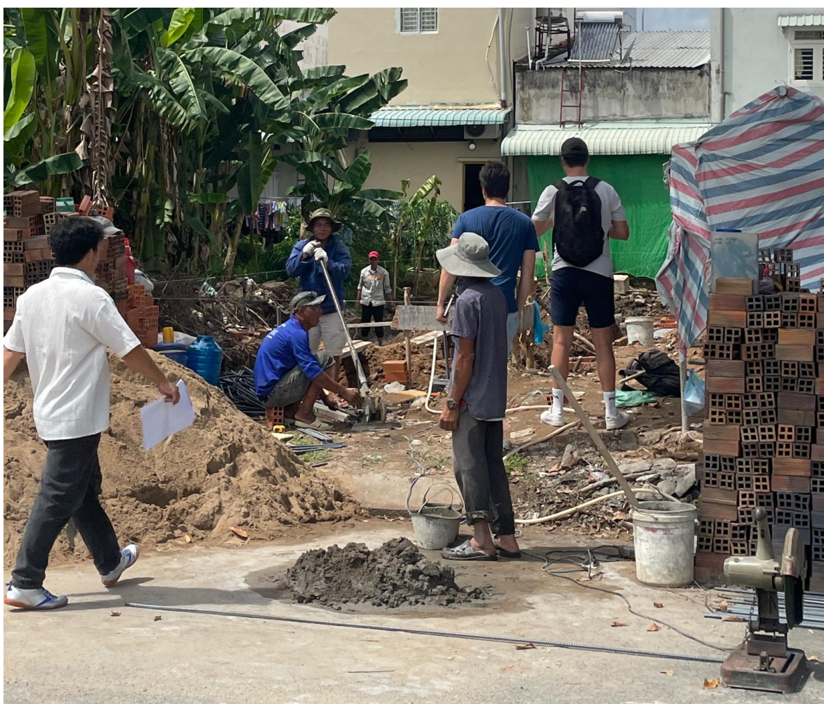
Figure 7.3: Installation of a fixed house (fieldwork 27 August 2024)
