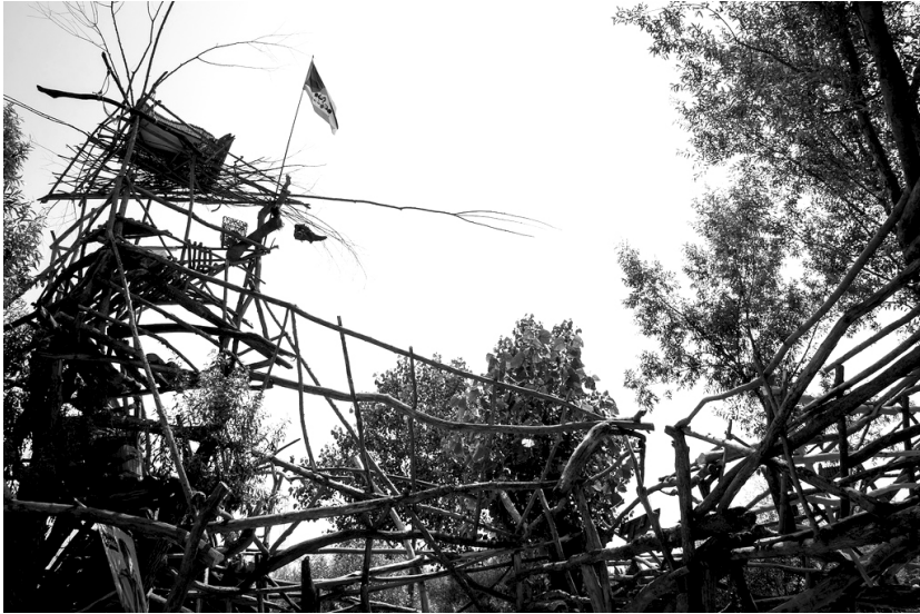
40 years structure along the Po River Alberto Manotti, Boretto, Emilia Romagna, Italy
