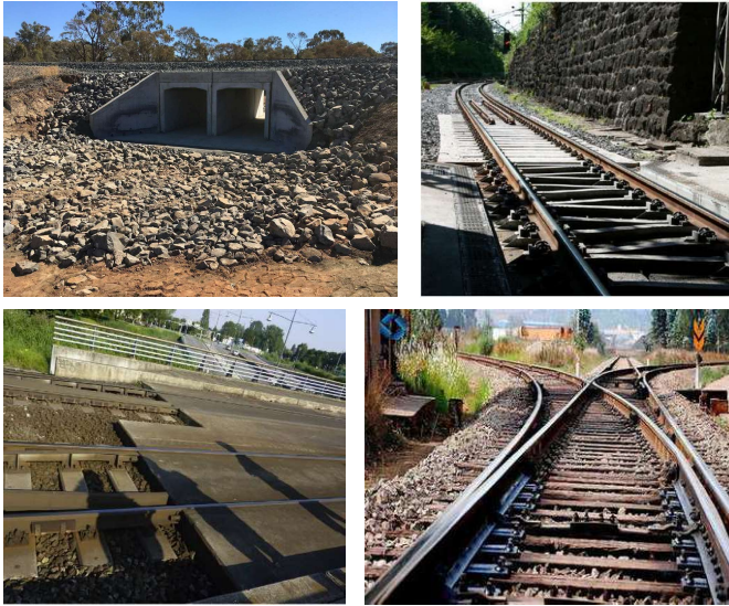
Figure 1.4: Different types of transition zones in railway tracks. Culvert (top left; source: https://joewagnergroup.com.au/projects/western-culverts-replacement/ ), tunnel (top right; source: [12]), bridge (bottom left; source: [4]), and switch (bottom right; source: http://www.railroadpart.com/rail-track-parts/railway-turnout.html ).
