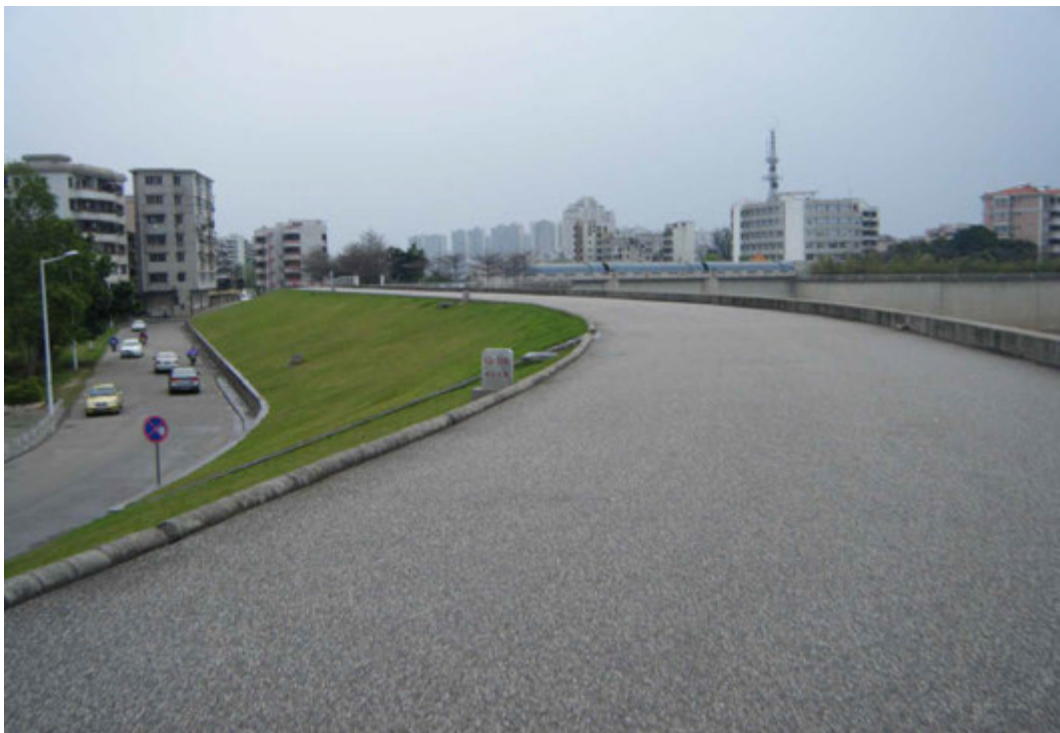
FIG. 2.17 The wide road on the Beijiang Dike was strictly controlled by the provincial water committee and not publicly accessible.
