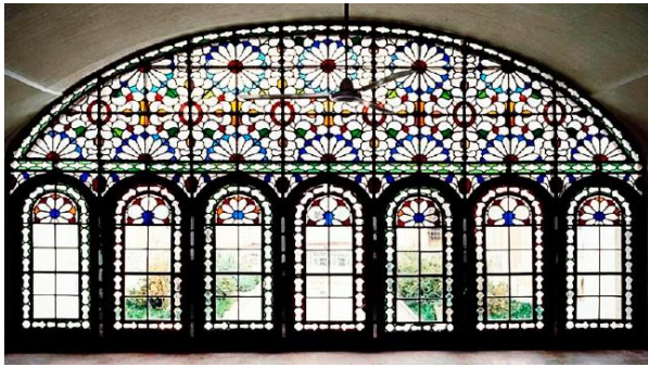
Figure 53: Windows facing courtyard Source: Sahebzadeh, Heidari, Kamelnia, & Baghbani, 2017
