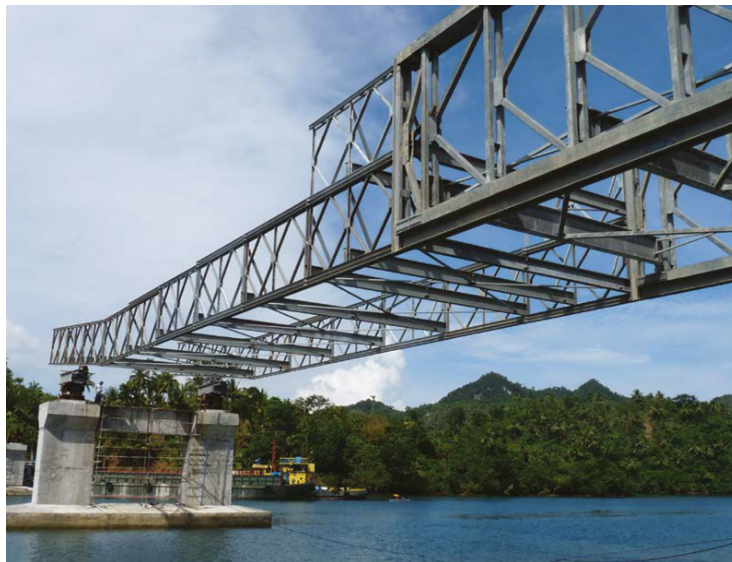
Figure 3.5: Variant of Mabey-Johnson bridge, showing differing panel size along span [32]
