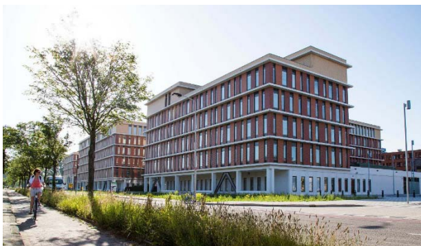
Figure 1. The exterior of the hospital.
