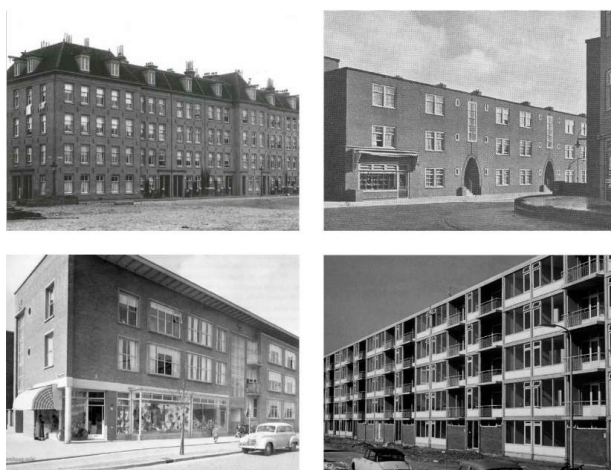
Figure 3. Four subtypes. Top left: subtype 1 interwar traditional construction methods Amsterdam. Top right: subtype 2 interwar traditional construction methods Den Haag. Bottom left: subtype 3 postwar mixed construction methods. Bottom right: subtype 4 postwar construction systems. Pictures are from the municipal picture data banks of Den Haag Amsterdam and Utrecht.
