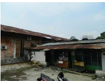
3. Newer Corridor Structure in between two buildings.
