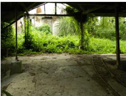
5. North Entrance to the inner yard.
