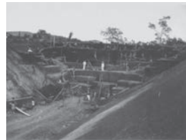
The making of railroad tracks around Purwakarta.
