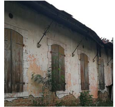
Outer part with tension rods that stabilize the light roof material (corrugated steel)
