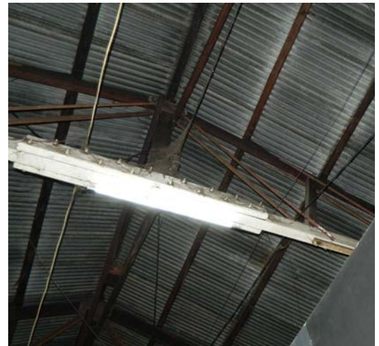
Existing roof structure with additional steel elements
