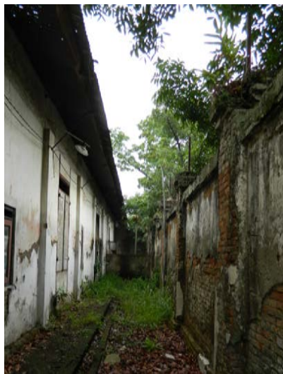
1. Back side of front Wall, South Elevation.
