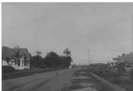
Housing construction on Jalan Riau which is still quiet.
