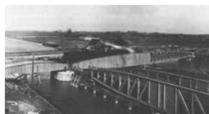
1907 Testing the new swing Bridge across the Gent0 Terneuzen Canal near Sluiskill
