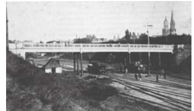
1868 Road bridge across the yard of the Rhenish Railway at Arnhem
