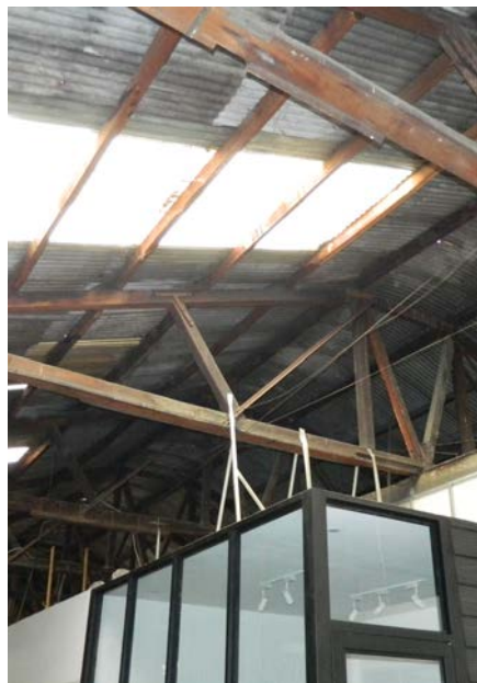
example of a building with visible roof structure and a row of supportive columns
