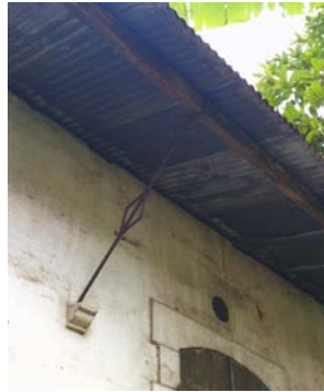
Outer part with tension rods that stabilize the light roof material (corrugated steel)
