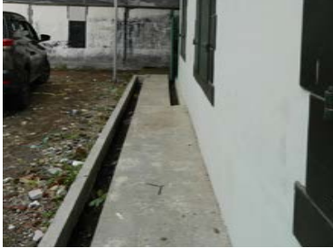
4. Building exterior corridor.
