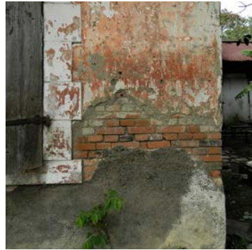
2. Arrangement of bricks in the corner
