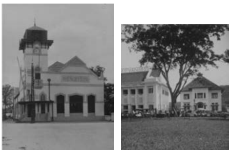
The establishment of banks in the Groote postweg is closely related to the rapid growth of plantation businesses around the city of Bandung and other efforts in the center of the city.
