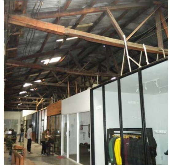
Existing roof structure with additional steel elements
