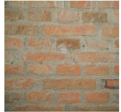
3. Part of the brick masonry wall of the building
