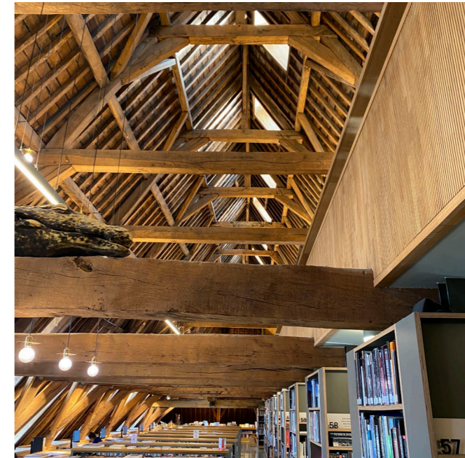
Exposed roof structure
