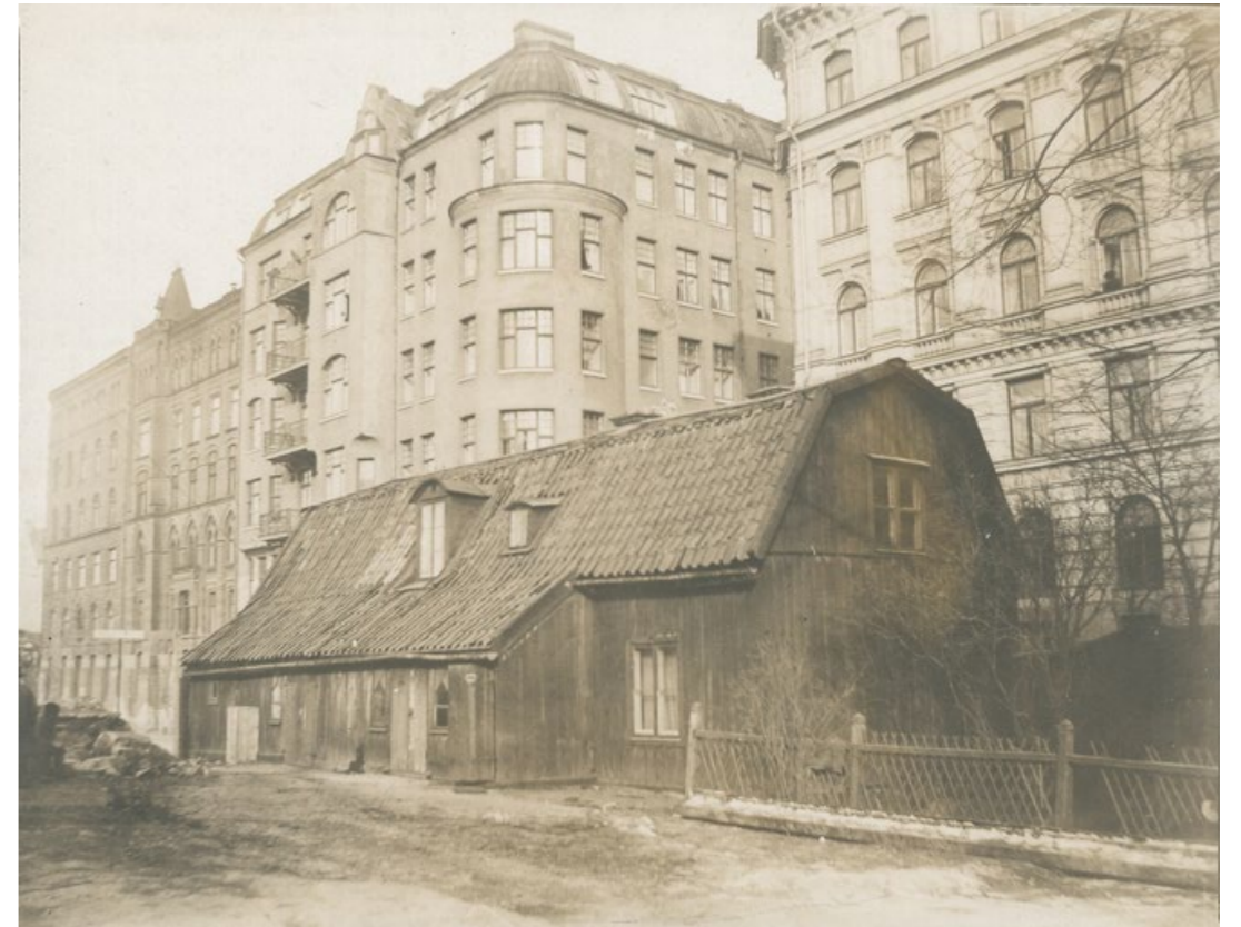
Sprängstensmur in the middle of the photo - traditional for the Swedish context Available at: https://www.bjornpatricks.com/BP2/Sveavaegen/Sveavaegen.html
