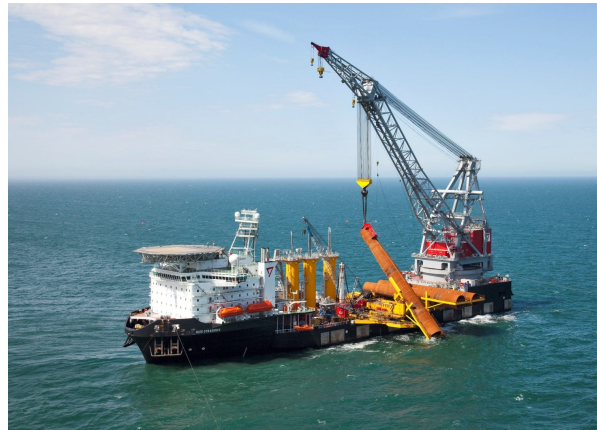
Figure 2.3: HLV Oleg Strashnov upending a monopile [15]
