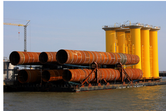
(b) Monopile transport on barge
