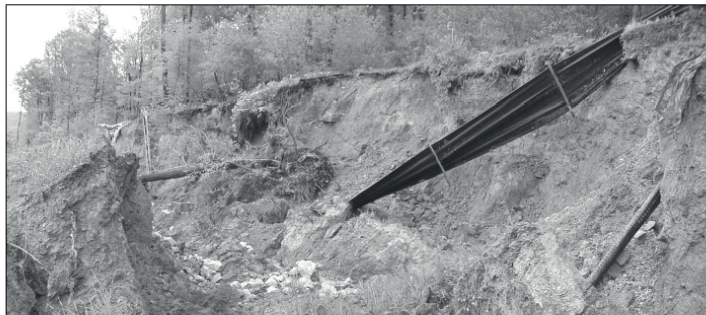
(b) View of 7.6 meter tall main scarp.
