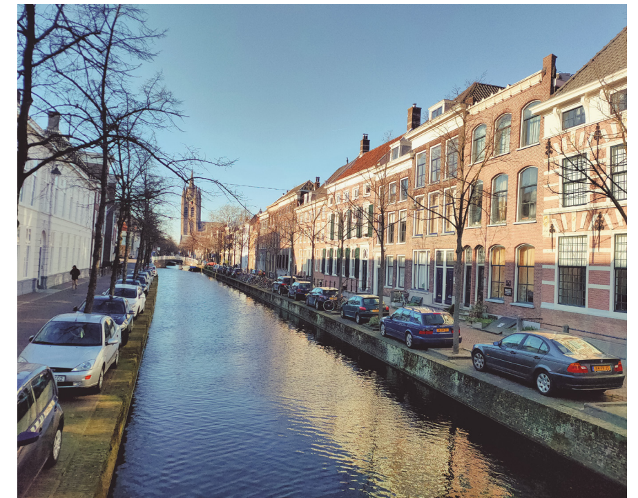
High quays lead to drowning hazards for hedgehogs, frogs and young swans.
