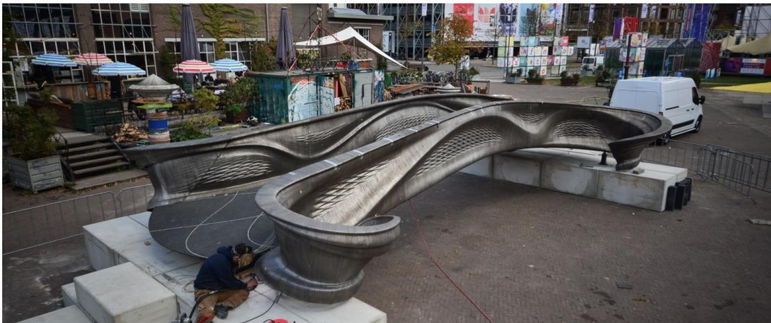
Figure 2.6: Additive manufactured bridge by MX3D
