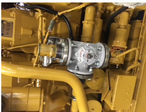
Figure A.9: Cooling three-way valve
