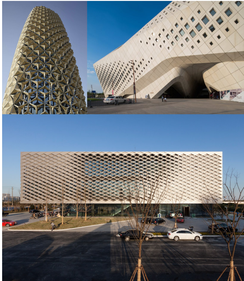
FIGURE 3.3 Recent examples of facades that follow a module-based approach. a. Al Bahar Towers, AEDAS, Image Credit: AEDAS; b. Nanjing International Youth Culture Centre, Zaha Hadid Architects, Image Credit: Khoo Guo Jie; c. Nantong Urban Planning Museum, Henn Architekten, Image Credit: Bartosz Kolonko/HENN
