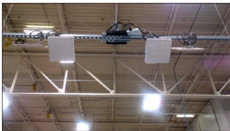
Figure B-5: RFID overhead reader - source: Mojix
