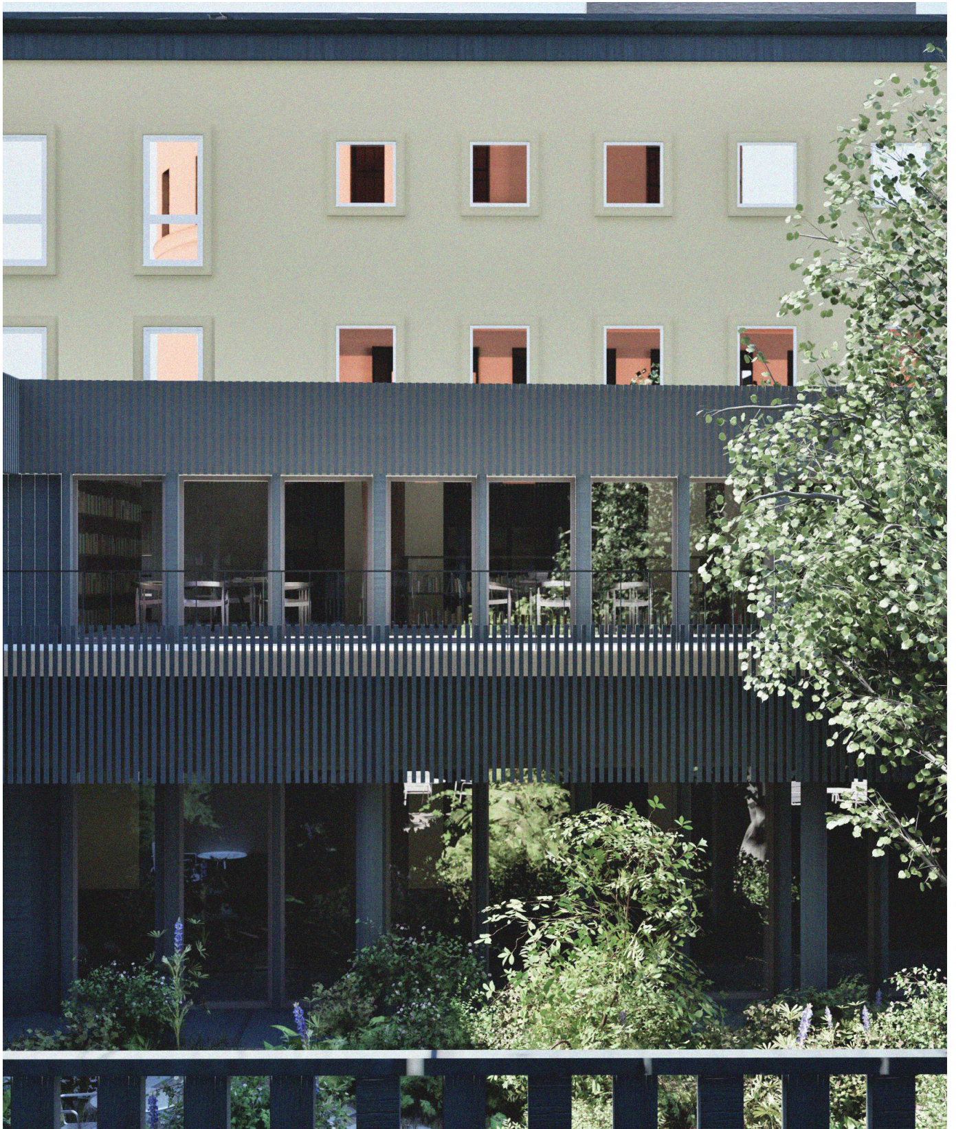
new visible link between the Library and the annex, through balconies
