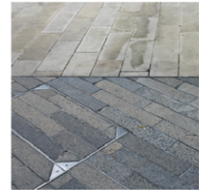
Material transitions No disruptions, clean and orderly
