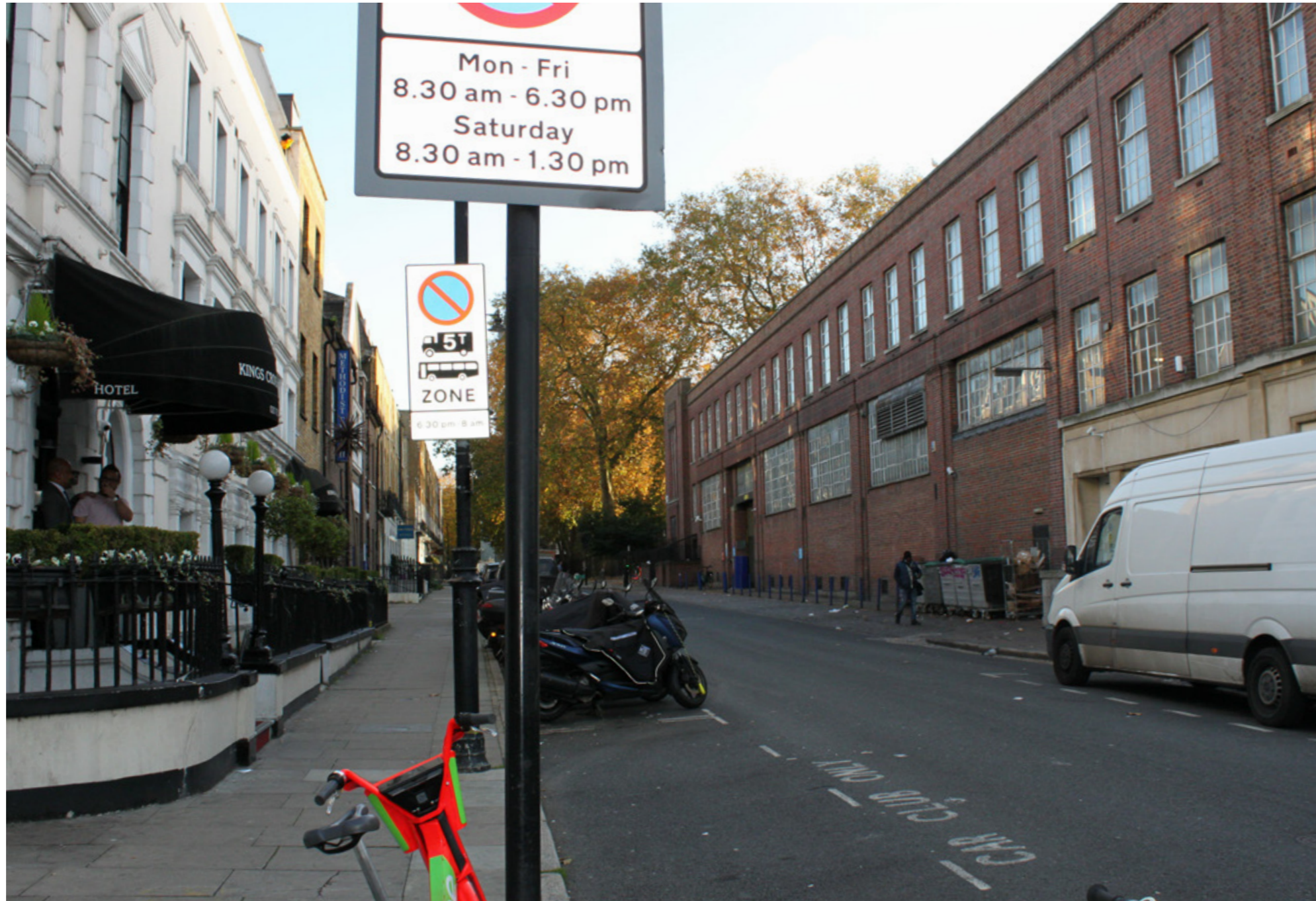
Belgrove House (right), currently in use by Access Self-storage
