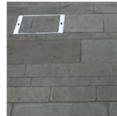
Metal details Clean and orderly, refined details
