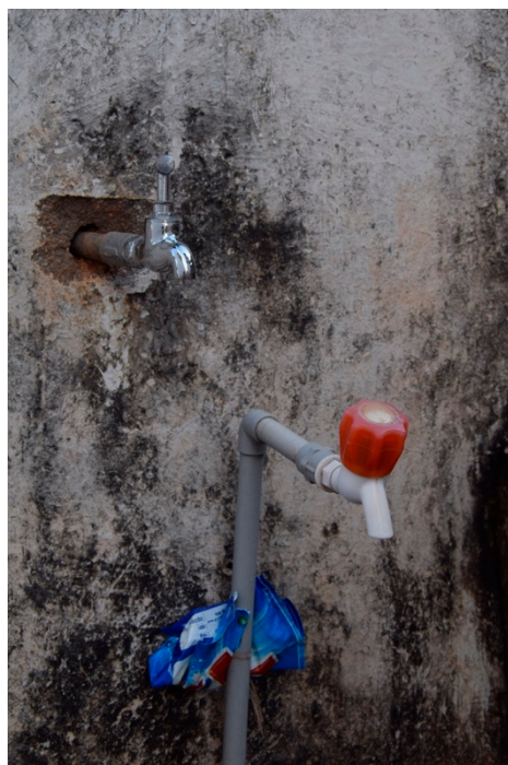
Figure 4. Two parallel supply systems—two water taps per household (photograph by C. Butsch).
