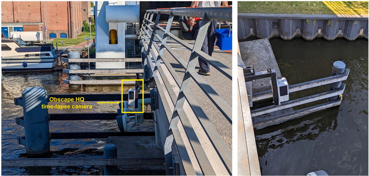
Fig. A.4. Monitoring setups at Groningen.
