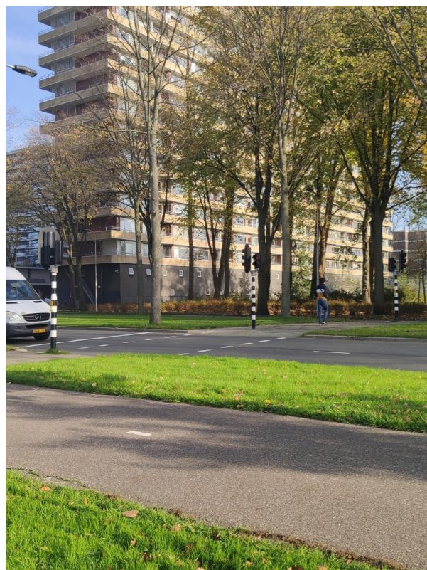
Figure 7 A cross walk controlled with traffic lights
