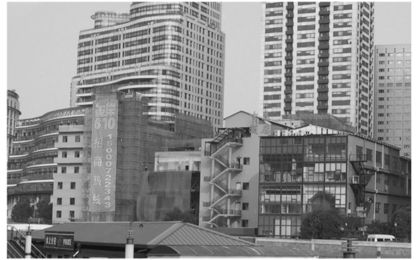
fig.04.2 (a) Existing Function in those Industrial Buildings (photo by author)
