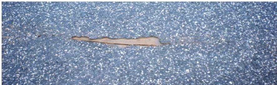
Figure 2.5: Visual observation of deck plate root crack [7].
