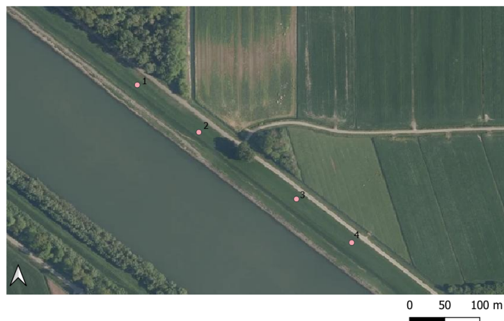
Figure 4.18: River dike section at the Amsterdam-Rhine canal. Between locations 1 and 2 conditions were normal. The area between locations 3 and 4 indicates the area which experienced wetting.
