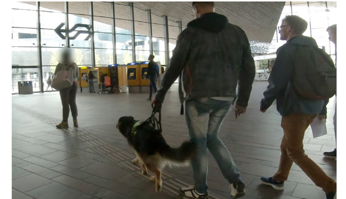
Fig 1.3- Obstructed tactile pavement in Rotterdam Central Station
