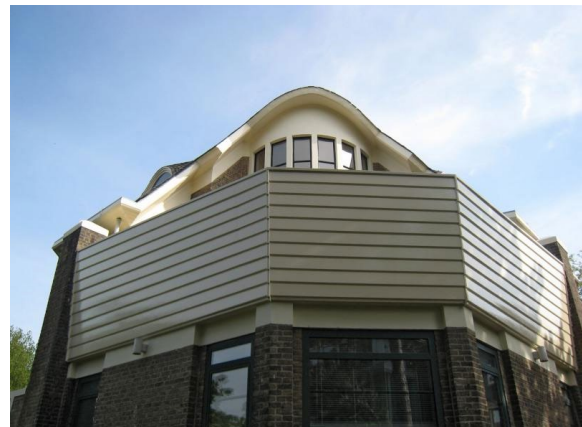
Image 20 Valentijn, D. 2009. Balcony east . Photograph. Den Haag: Monumentenzorg.
