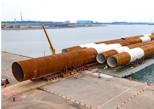
Figure 5.18: Transportation of monopiles on a barge [77]
