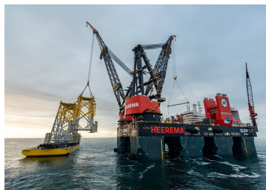
Figure 5.21: Installing a jacket [80]
