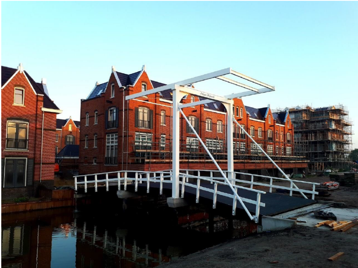
Figure A9: Rhijngeest bridge, Oegstgeest (Dura Vermeer, 2020c)
