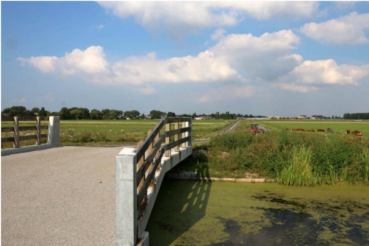
Figure A7: Bridge Schiebroeksepolder, Schieveen (Midden-Delfland, 2019)
