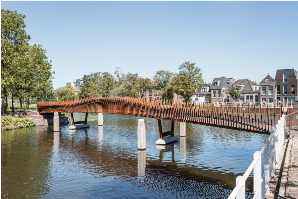
Figure A8: Wisenniabrug, Leiden (Ney & Partners, 2020)
