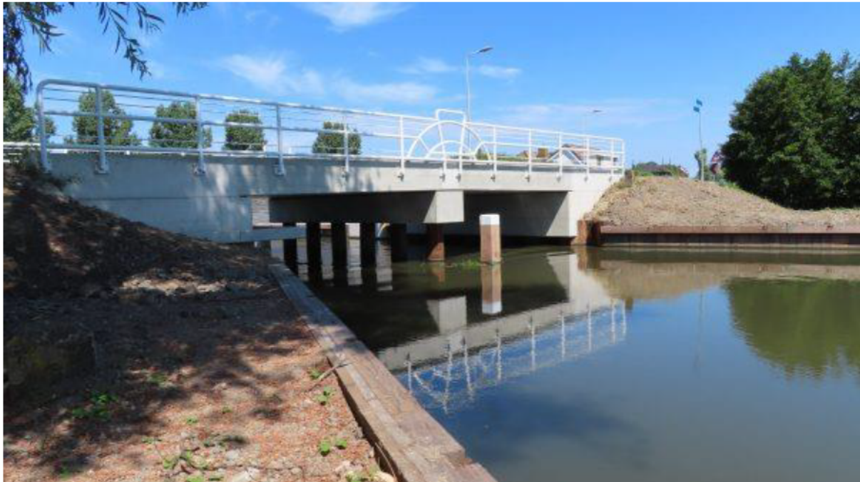
Figure A6: Traffic bridge Enkele Wiericke, Nieuwerbrug (BR6, 2022).
