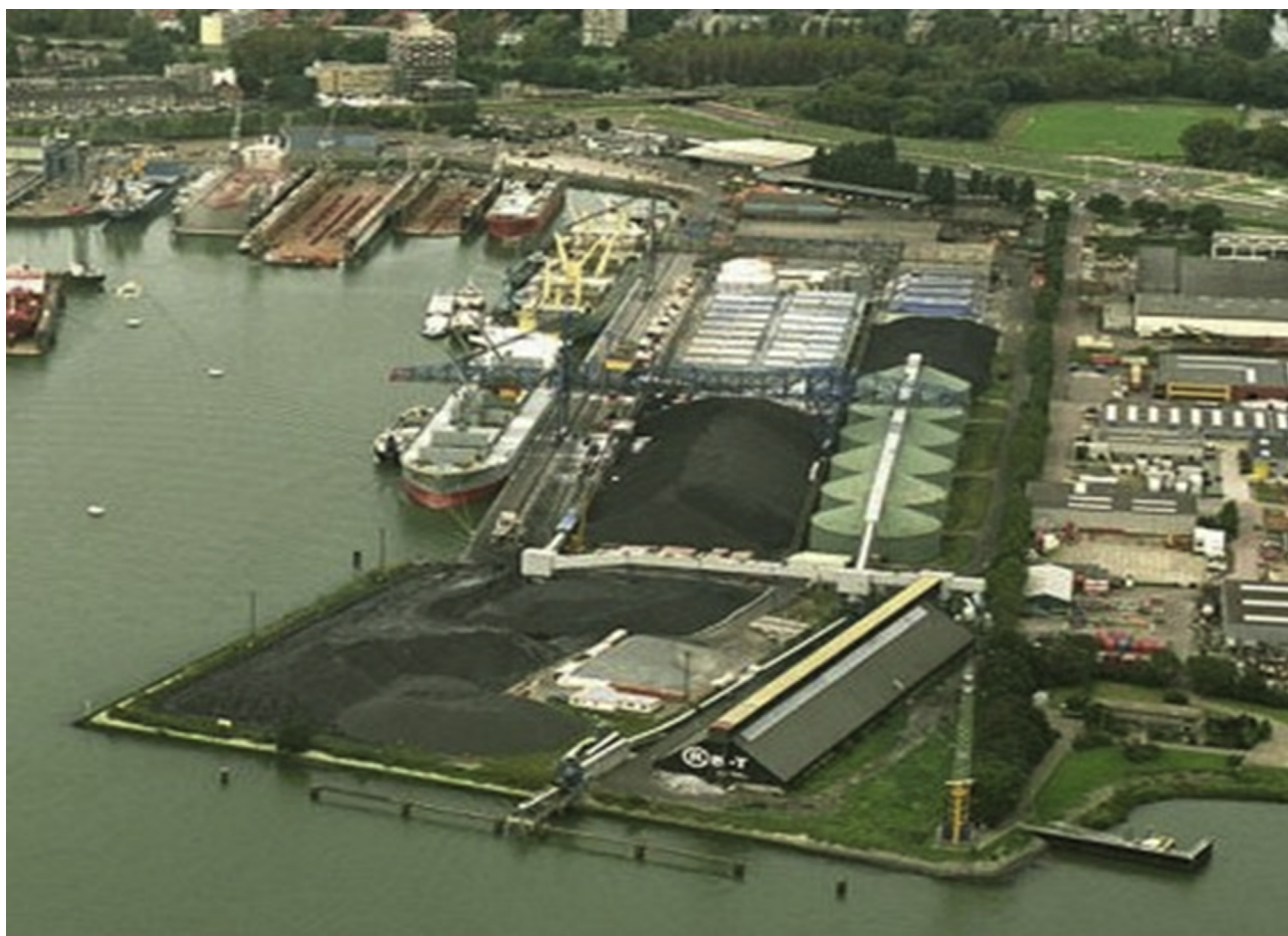
Fig. 15. Rotterdam Bulk Terminal aerial view (Image courtesy of RBT BV).
