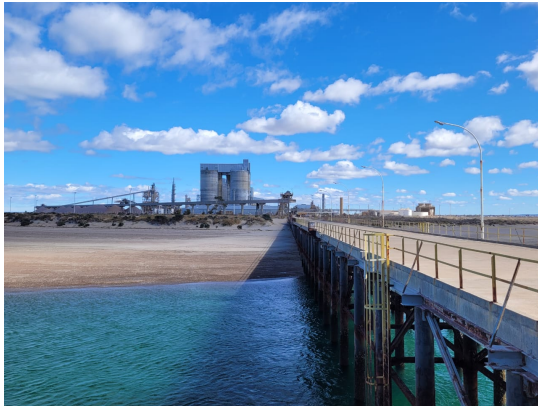
(a) The pier, facing the ALPAT plant
