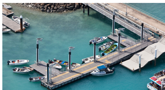
Figure D.6: Example of a piled pontoon marina ( TJS Marine - Floating Pontoons , n.d.)
