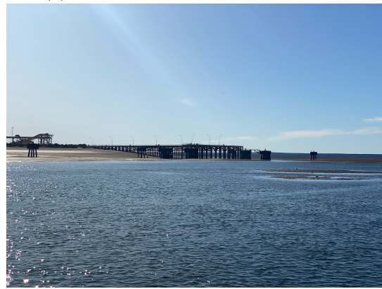
(d) The pier during low tide, picture taken from a boat
