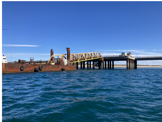
Figure D.8: Example of a combination of a fixed pier and a floating pontoon, SAE pier
