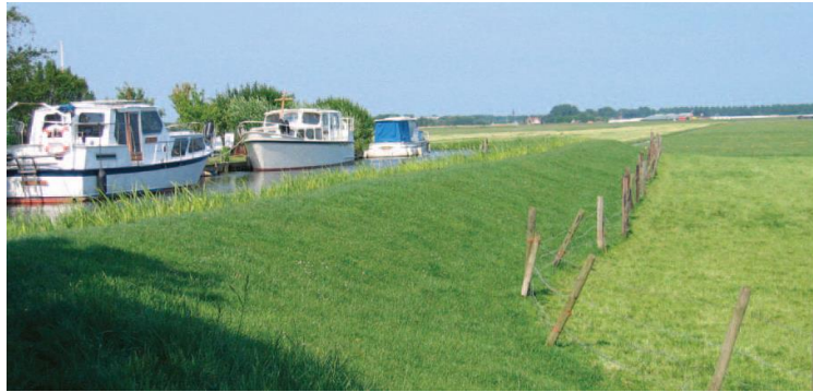
Figure 4-3. Example of canals in Rijnland, where the water level is higher than the surrounding fields
