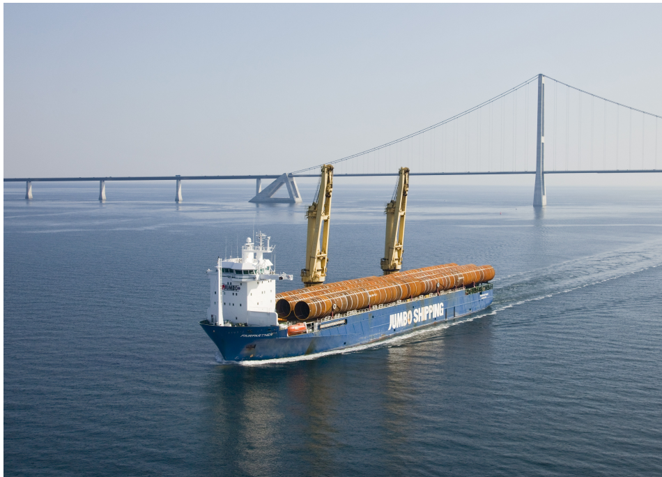
Figure 2.2: A transportation vessel transporting the monopiles to the wind farm location. Some HLVs can carry the monopiles on deck. Other means of transportation are using barges or wet-towing the monopiles. 0
