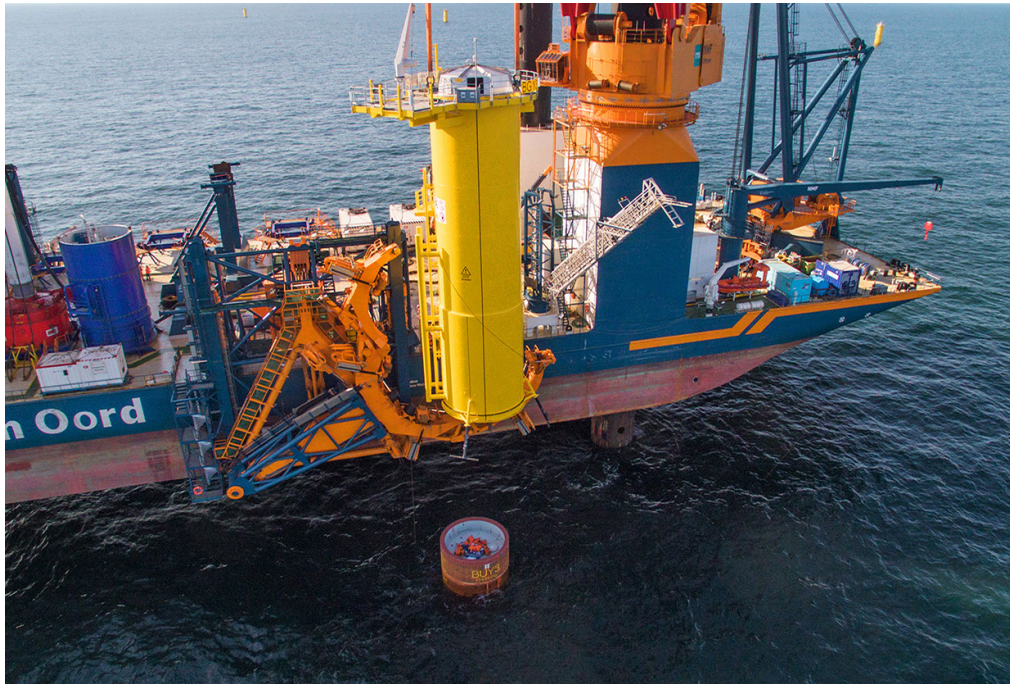
Figure 2.5: A transition piece being installed onto the monopile. [9]
