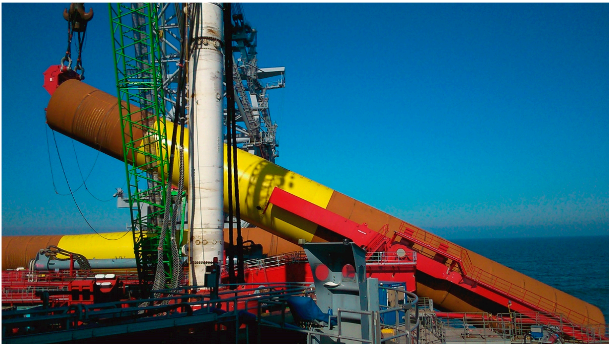
Figure 2.3: An example of an upending tool with a capacity of 1,400 tonnes that clamps the monopile at the top. 1
