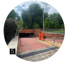
Underground parking lot
