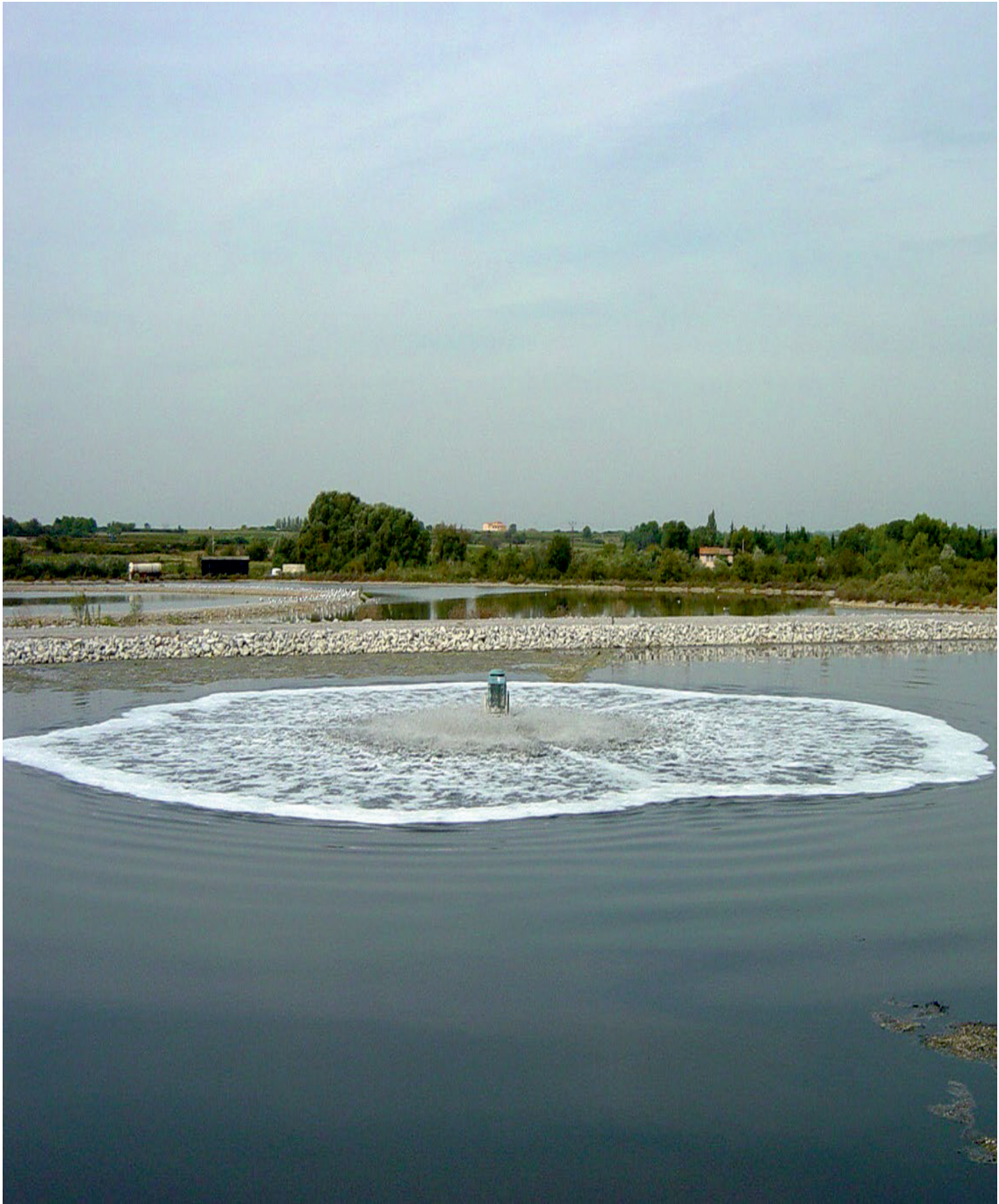
Aerobic lagoons and ponds are in many low- and medium-income countries prevailing technologies for the removal of organic matter from sewage, and faecal and septic sludge, often in combination with anaerobic and facultative ponds (photo: M. von Sperling).
