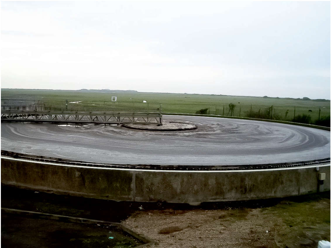
Extreme manifestation of sludge bulking in a secondary settler (photo: D. Brdjanovic).
