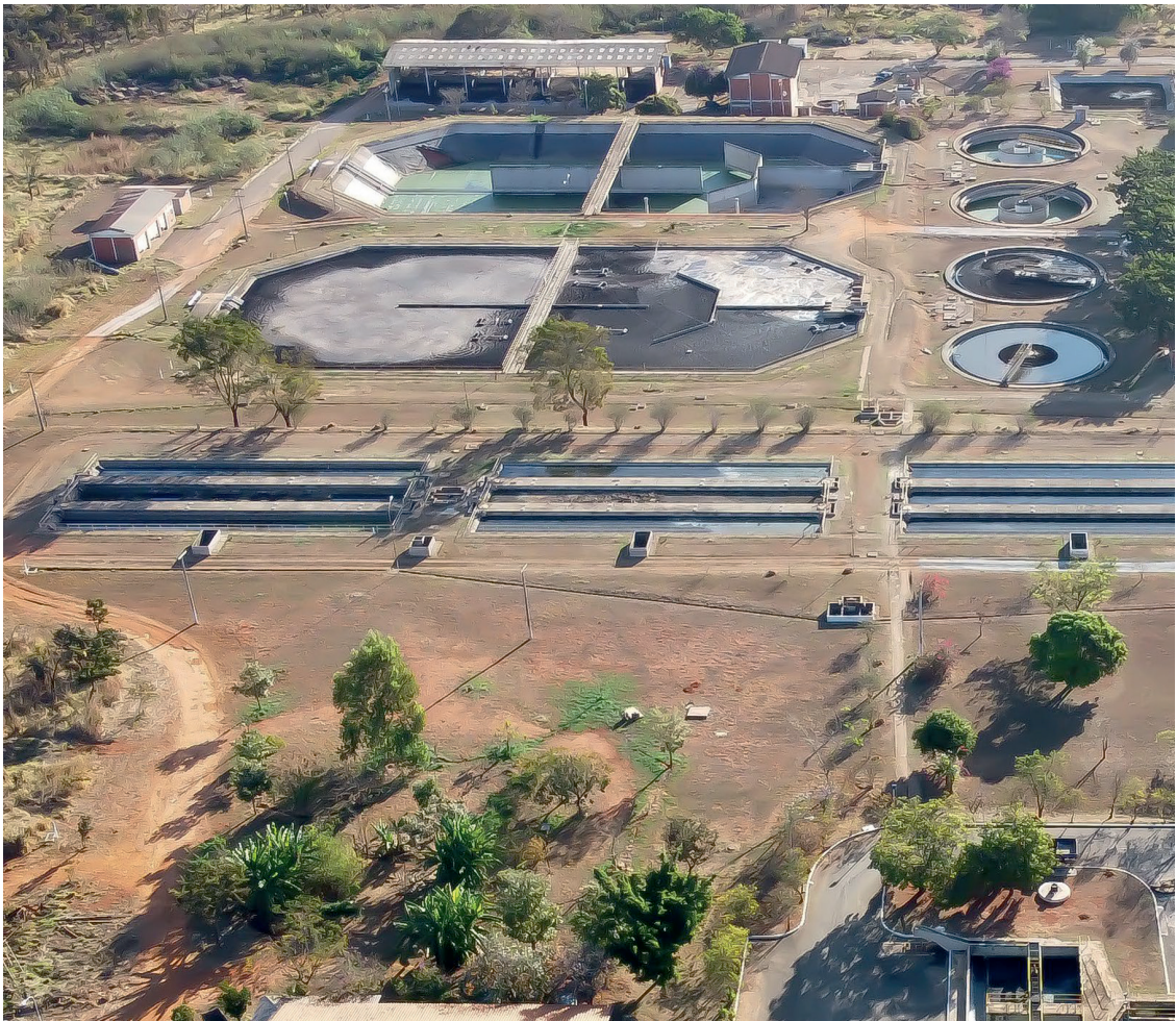
WWTP plant Gama in Brazil – an example of a 5-stage Bardenpho process for the removal of organic matter, nitrogen and phosphorus (photo: G. Da Luz Lima Júnior).
