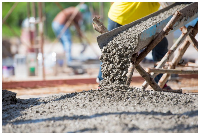
Figure 1: Pouring concrete on site (GCP, 2018)
