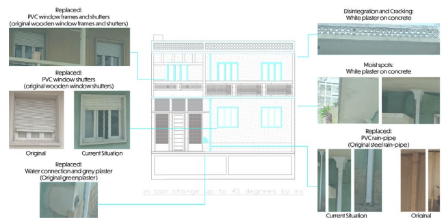
Figure 7: Front Façade with assessed damage
