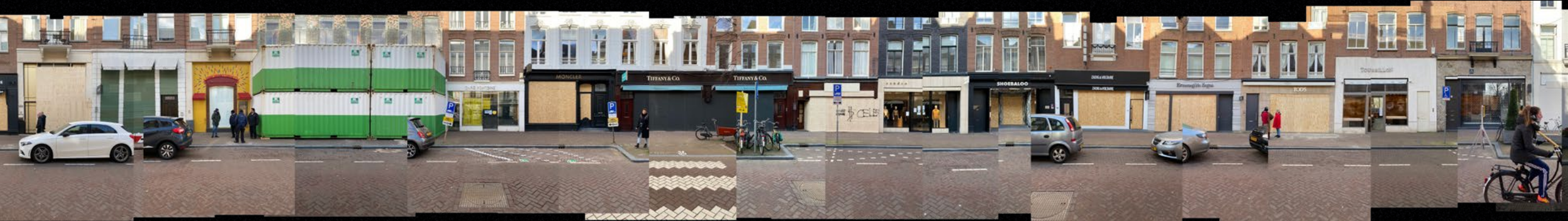
P.C. HOOFSTRAAT (NORTH SIDE) AMSTERDAM, THE NETHERLANDS P.C. Hoofstraat, Amsterdam, in lock-down on January 31st 2021. To prevent vandalism and destruction by riots that took place in that neighbourhood at that time, the closed luxury stores transformed into temporary fortresses.
