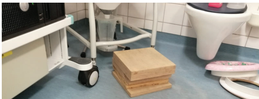
Image 2.4. ErasmusMC's solution to different leg lengths among kids using the same toilet.
