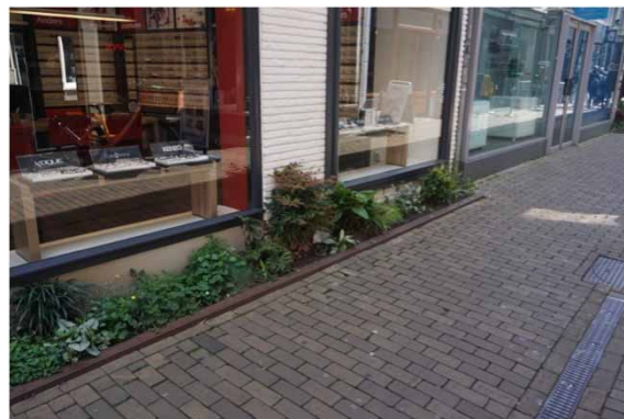
Figure 3 | Case #30: a facade garden, which has been assigned the root cause embedded practices of involved actors. A facade garden is typically constructed surrounded by raised borders. Preventing runoff to be drained into the garden, this reduces the effectiveness of the SUDS.
