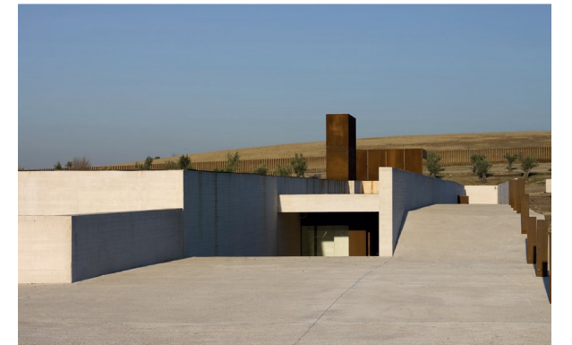
Use of white concrete and rusted steel i.e. contemporary materials that communicate with stucco and ceramic of the ancient city.
