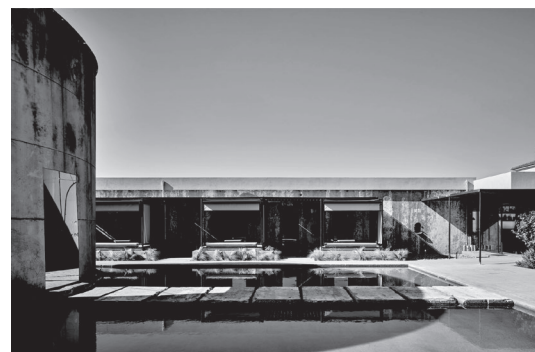
Concrete blocks divided for wine storage tanks (5m x 6m) used as hotel rooms. Doorway openings - slabs used as stepping pathway.
