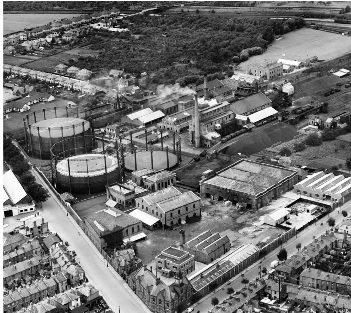
1800-1900: Functional Pieces of Engineering Prime locations to deliver gas/electricity to the area
