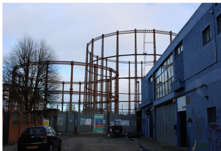
View from Marian Place Gasholder No. 2 and 5 seen from the previously used main entrance of the gas storage station site
