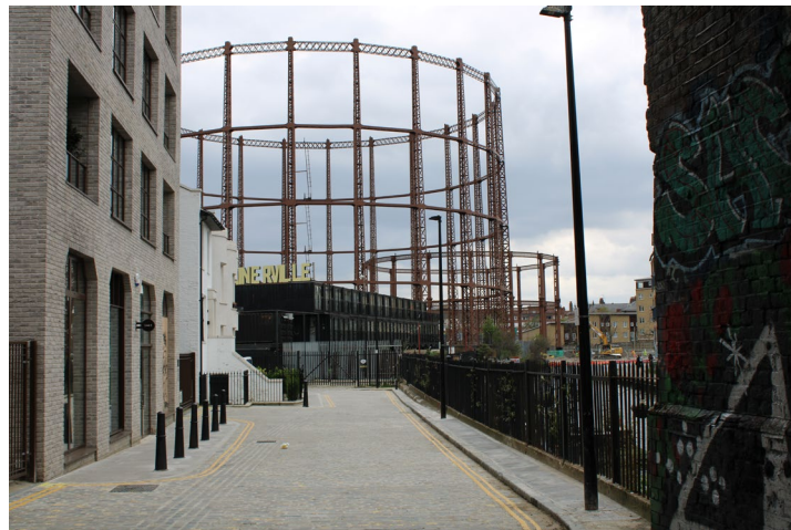
View from Corbridge Crescent Prominent view of the gasholders, framed by the tunnel and the railroad bridge above
