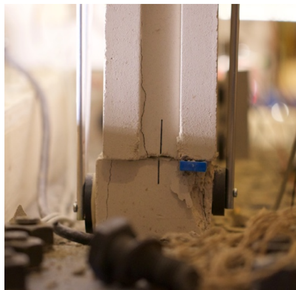
Figure 7. Out-of-plane displacement of element 8 in wide pier 3.
