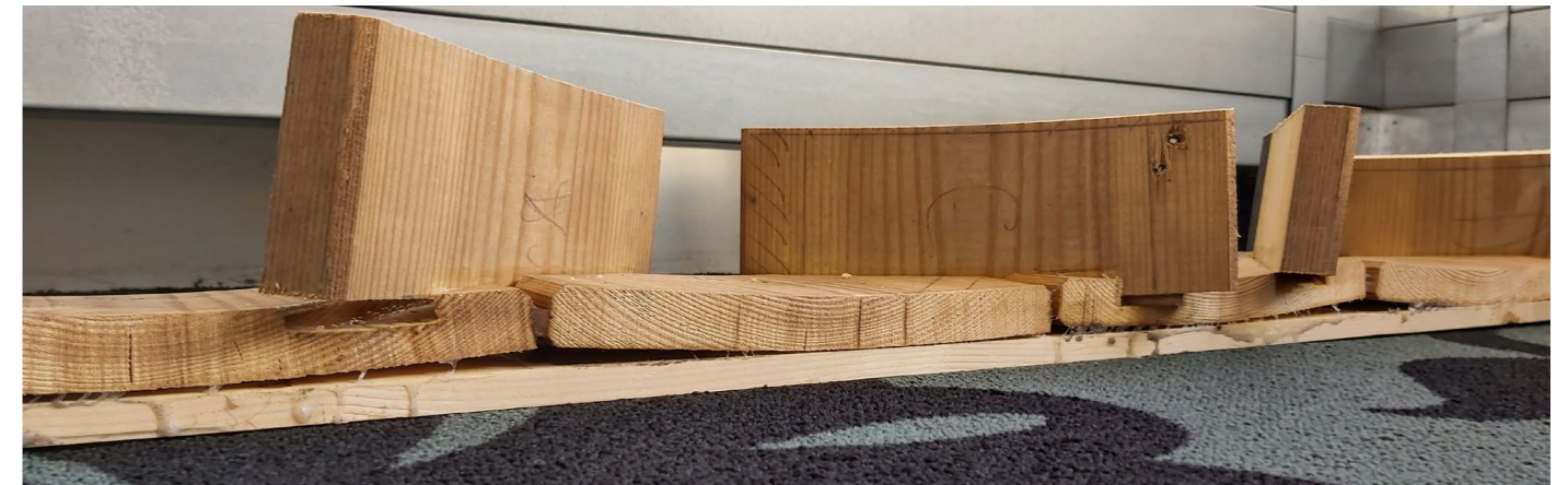
Figure 67: Detached elements due to excessive curving.
