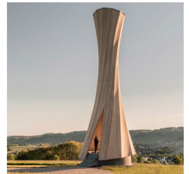
Figure 19: The Urbach tower. (ICD/ITKE University of Stuttgart., 2019)
