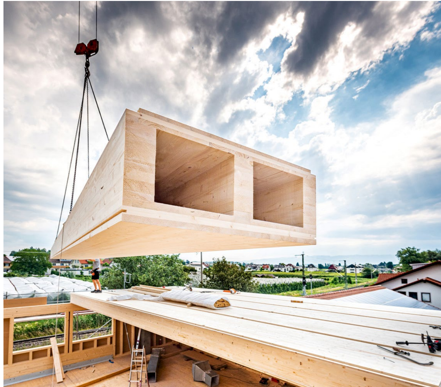
Figure 40: CLT boxfloor element. (Best wood Schneider, n.d.)
