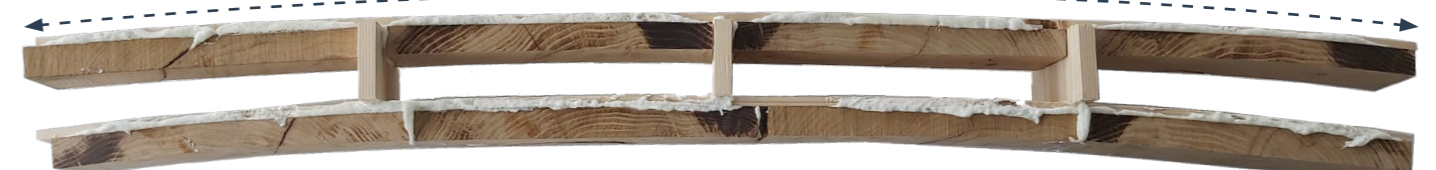
Figure 77: Increased curvature after significant 'drying'-time.
