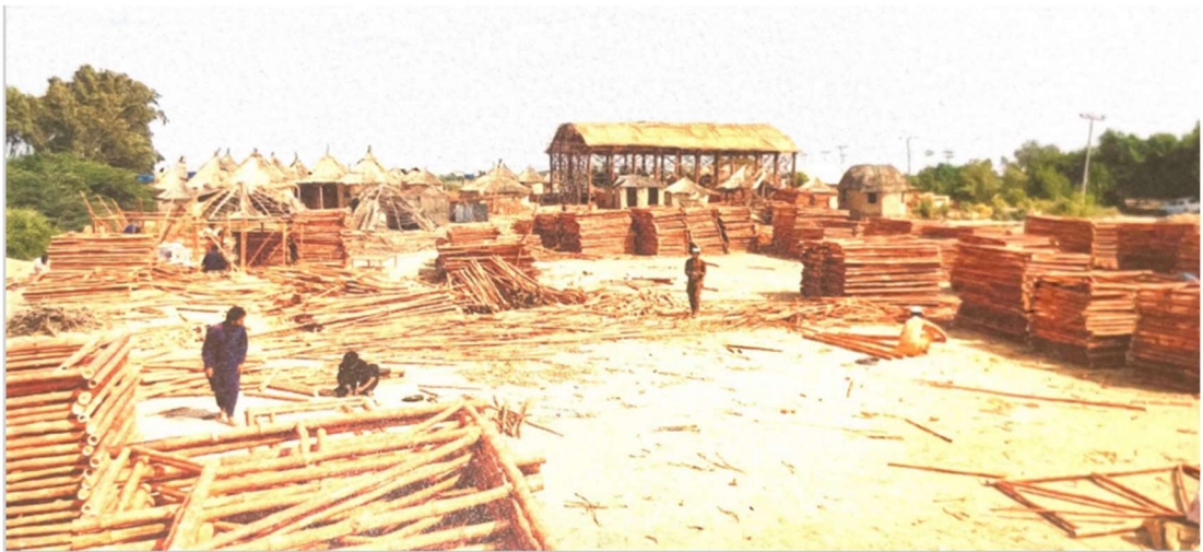
The pre fabrication of the bamboo modules, 2022, (Fitz, 127)
